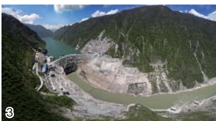
3. Jinping Phase-I Hydro Power Station has a 305 meters-high arch dam, the highest in the world. 4. Tianjin SDIC Jinneng Electric Power Co., Ltd. is a “Five-in-One” project of circular economy, consisting of power generation, sea water desalination, salt-making from concentrated sea water, land reservation and consolidation and reusing of the waste. 5. SDIC Shizuishan Solar Power Co., Ltd. has a total installed capacity of 45MW. 6. SDIC Baiyin Wind Power Co., Ltd. is SDIC’s first wind power company.
