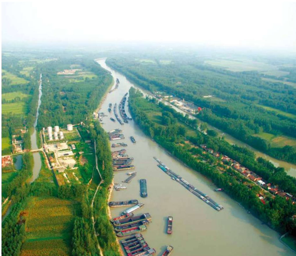
Skyview von Canal Suqian Port
