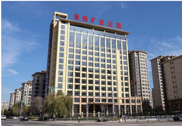
Shandong Energy Luxi Mine Industry Co.,Ltd.
